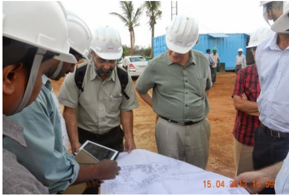
ICTS under construction, April 2013
