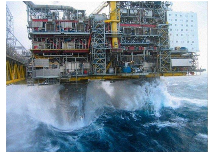
Wave impacting the deck underside (Abdussamie, 2016)
