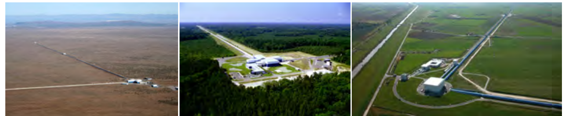
Fig. 2: LIGO Hanford (left), LIGO Livingston (middle) and Virgo (right) interferometers. LIGO detectors both have 4km arms while Virgo has 3km arms.
