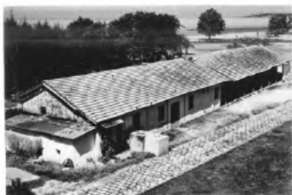
Old Military Hutments on the Colaba site being used as laboratories during the construction of the buildings.
